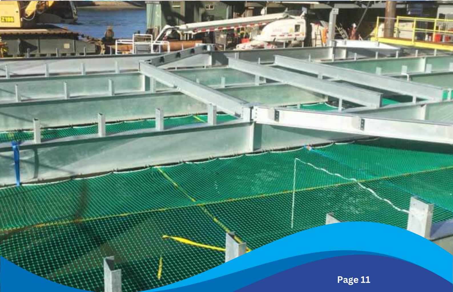
Photos of a System S Safety Net at Howard Street Wharves - Brisbane
